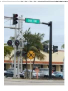
**Project Description:** This project is for the refurbishment of the traffic signal mast arm assemblies that have deteriorated. Scope of work includes stripping existing paint, priming, painting black, and required maintenance of traffic for thirteen (13) intersections with mast arms. Project also includes the vinyl wrapping of 80 traffic signal control boxes with artwork. During FY 2016, the City painted and treated several mast arms on Dixie Highway.
