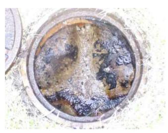
**Project Description:** This project involves the rehabilitation of deteriorated brick manholes located throughout the City. Rehabilitation consists of covering the interior surfaces with an adhesive, non-permeable material. 108 manholes were lined in FY15 and FY16. Citywide there are 4,400 manholes.
