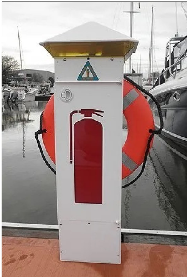
TYPICAL FIRE EXTINGUISHER CABINET STAINLESS STEEL POWDER COATED WHITE 10LB EXTINGUISHER LIGHT & ALARM OPTIONAL SUPPLIED BY MARINA ELECTRICAL EQUIPMENT, EATON CORPORATION, OR APPROVED EQUAL
