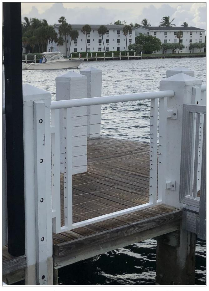
EXISTING ALUMINUM W/ STAINLESS STEEL CABLE RAIL SYSTEM (CONTRACTOR TO MATCH FOR RAILS ON THE WATER TAXI DOCK, FISHING PIER EXTENSION & RAILS ALONG TOP OF BULKHEAD. ALL OTHER RAILS PER DETAILS PROVIDED, HEREIN.
