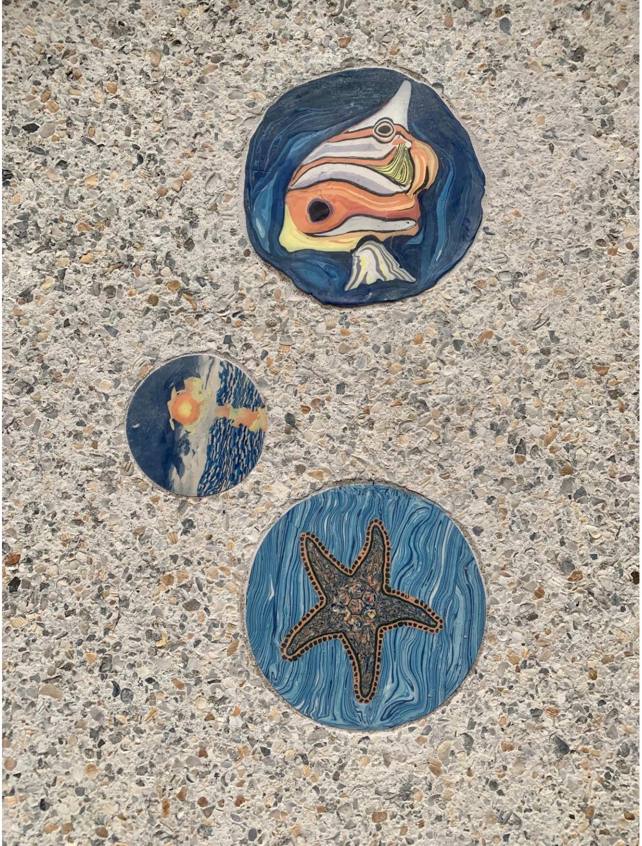
The Beach Mosaic Team Term 2: SEA LIFE By Sonata Kazimieraitiene 99 Hand-made Tiles. Installed 2022.
