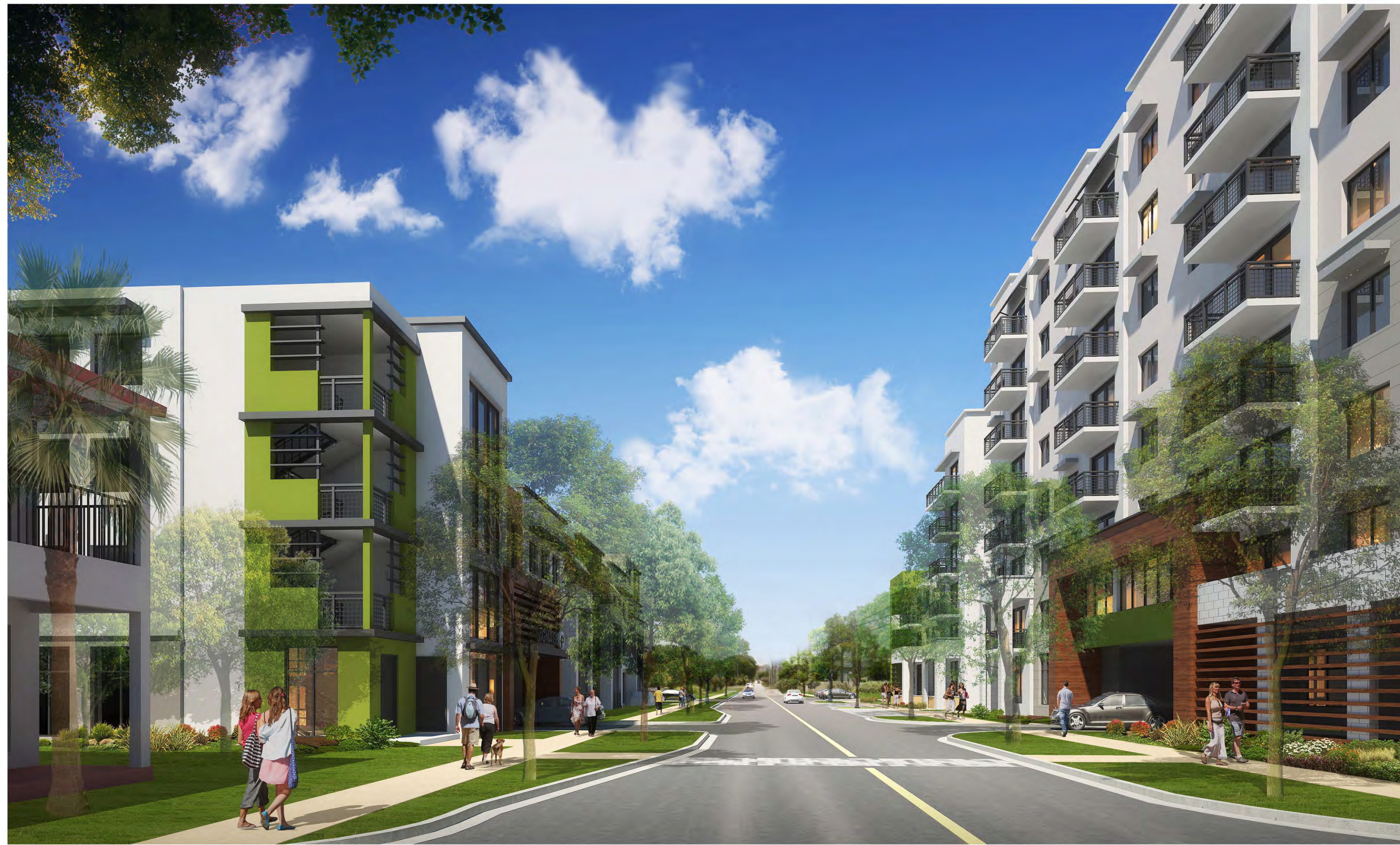
5 VIEW LOOKING WEST FROM 16TH ST
