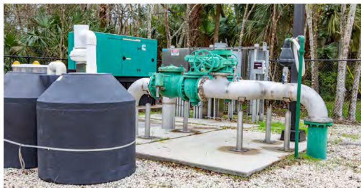
► City of Palm Coast - Lift Station D Improvements
