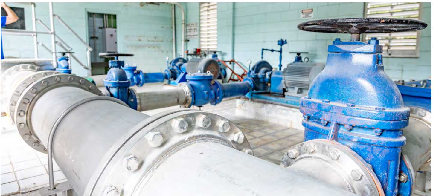
► City of Palm Coast - Pump Header Replacement
