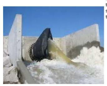
**Project Description:** This project is to install check valves on tidal outfalls. The valve will prevent backflow of tide onto streets during extreme high tides, when tidal waters are higher than the roadway.
