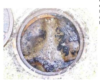
**Project Description:** This project involves the rehabilitation of deteriorated brick manholes located throughout the City. Rehabilitation consists of covering the interior surfaces with an adhesive, non-permeable material. 108 manholes were lined in FY15 and FY16. Citywide there are 4,400 manholes.
