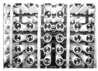
**Project Description:** This ongoing project consists of replacing the membrane elements when needed. The membrane elements are used to purify water to make it potable and requires replacement every 5 years. Funding will be budgeted over a multi-year period to provide for full replacement.
