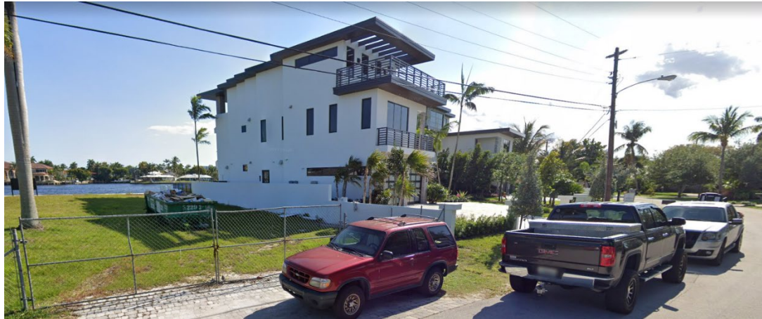
View of retaining wall from adjacent vacant lot
