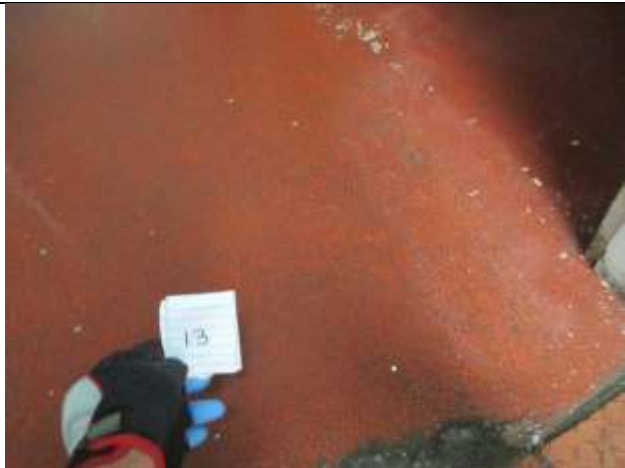
HA 13- Red Rolled Sheet Flooring and Glue
