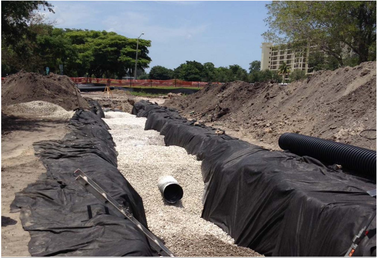
NEW DRAINAGE INSTALLATION
