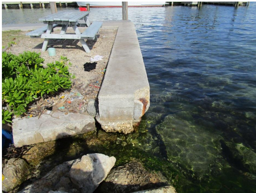
Plate D North View at East End along ICWW. Major crack / loss of concrete and spalling corner.
