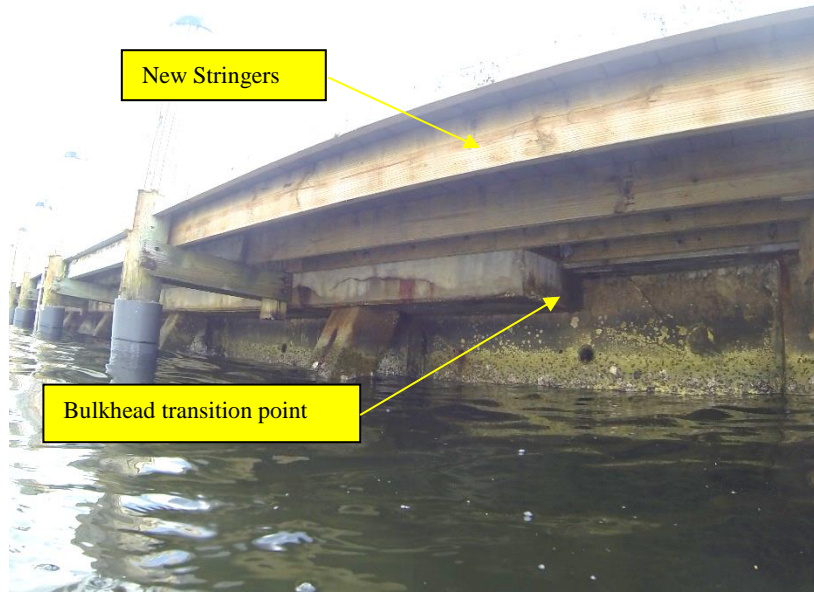
Plate O View beneath dock at bulkhead transition point Note repaired section of timber dock
