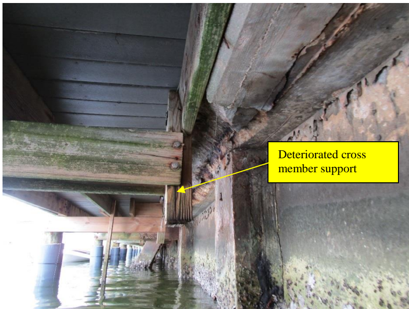
Plate T Typical condition of bulkhead cap and dock
