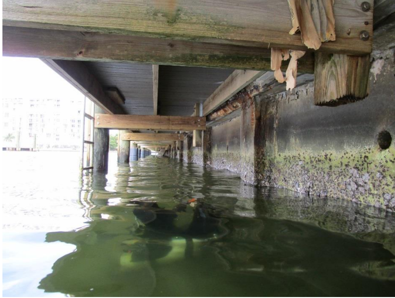
Plate S Typical condition of bulkhead cap and dock
