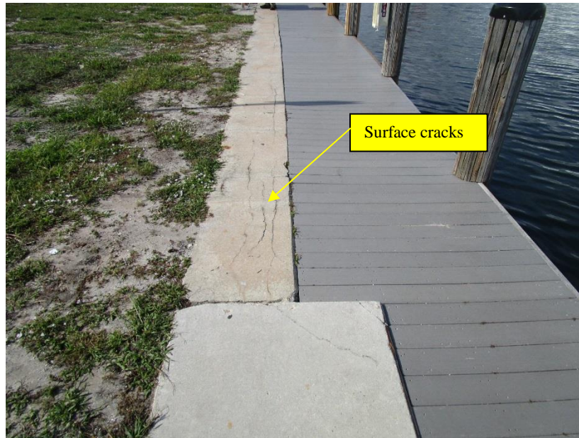
Plate K West view at transition from repaired bulkhead section to original bulkhead structure
