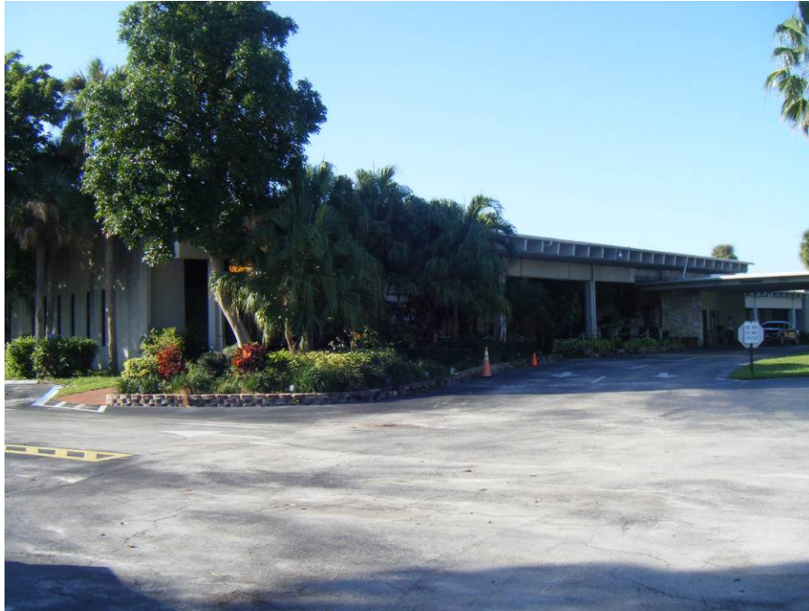
FRONT VIEW OF CLUBHOUSE
