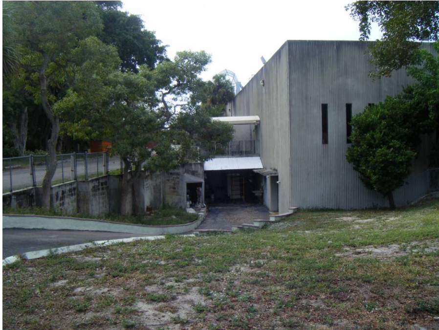
BASEMENT ENTRY TO CLUBHOUSE
