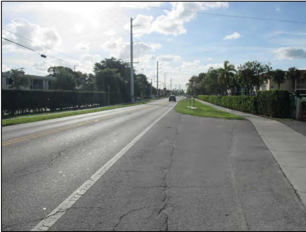
LOOKING WEST ALONG EAST MCNAB ROAD WITH SUBJECT AT RIGHT
