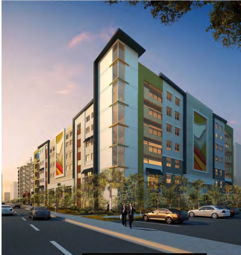
VIEW OF GARAGE HEADING N
