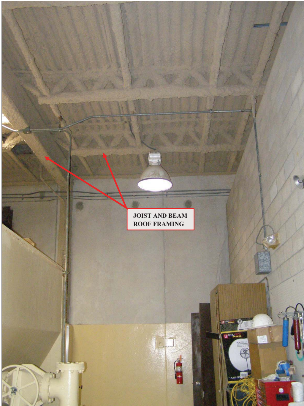
Photo 30: Typical Roof Framing
