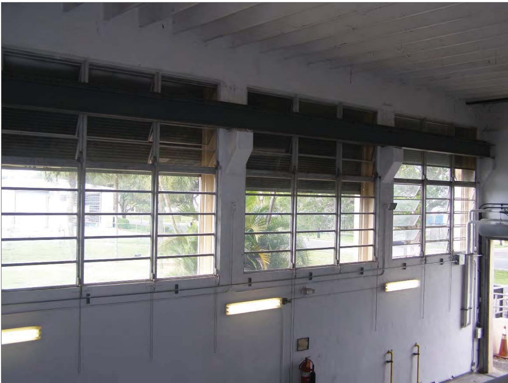
Photo 4: Interior View of Windows
