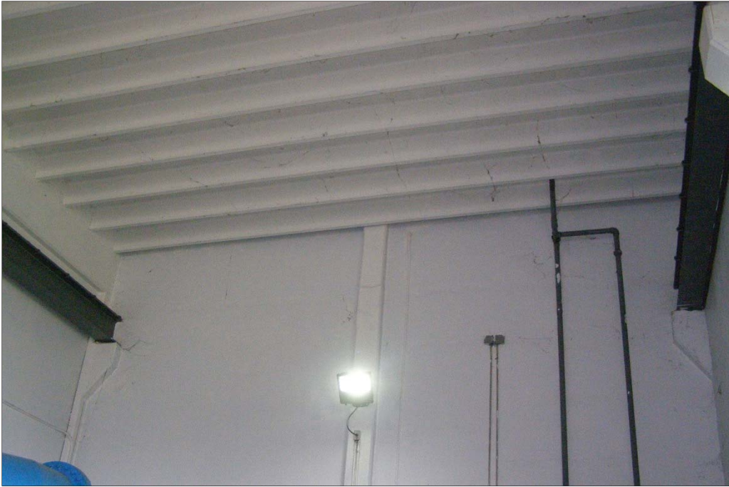
Photo 3: Typical Double Tee Roof Structure
