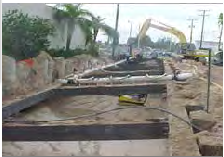
Renaissance 72" Aluminized Steel Pipe (20' deep)
