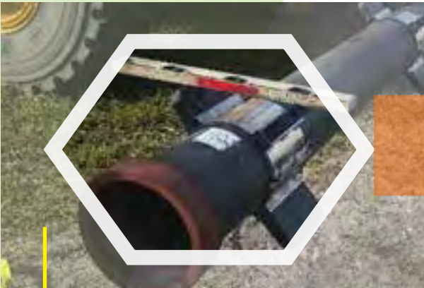
Pipe Spacers in Place for Casing Installation
