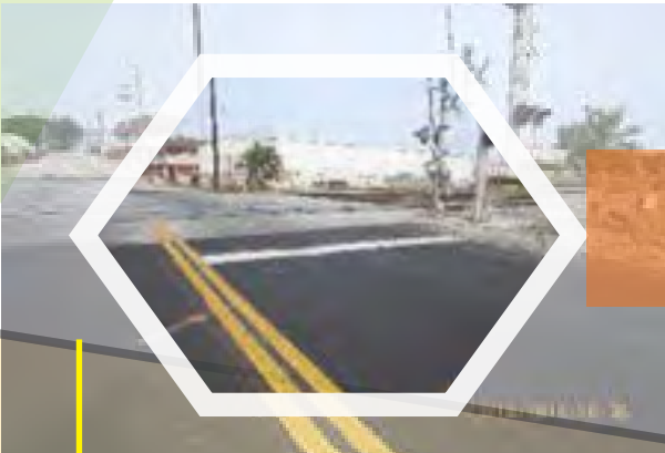
Jack & Bore Completed
