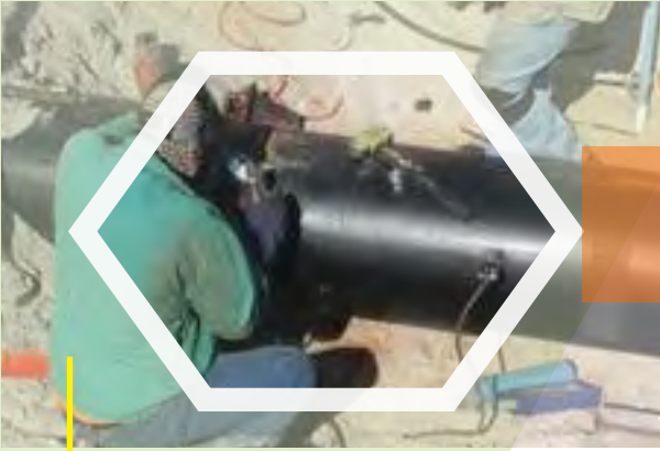
Welding Pipe Casing
