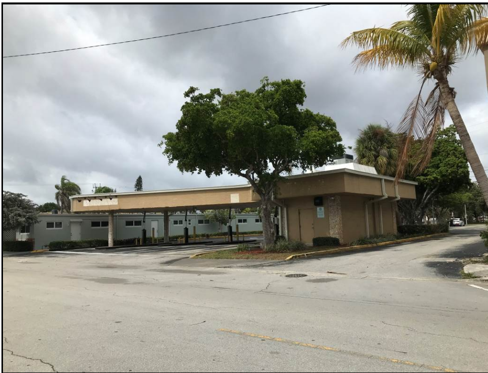
VIEW OF SUBJECT PROPERTY FACING SOUTHWEST
