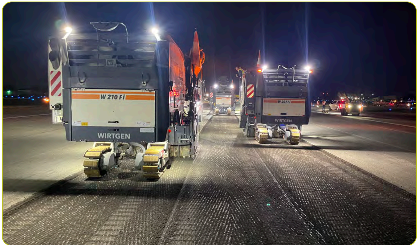
FXE Runway 9-27 Pavement Rehabilitation
