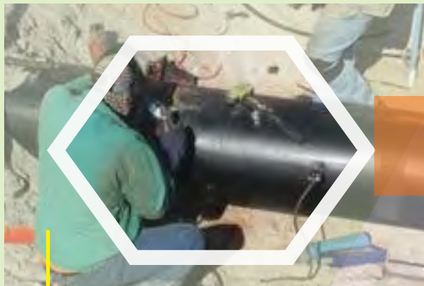
Welding Pipe Casing
