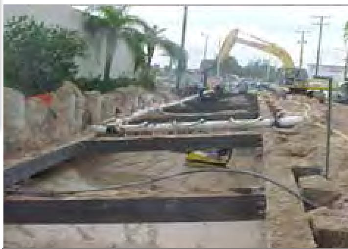
Renaissance 72" Aluminized Steel Pipe (20' deep)
