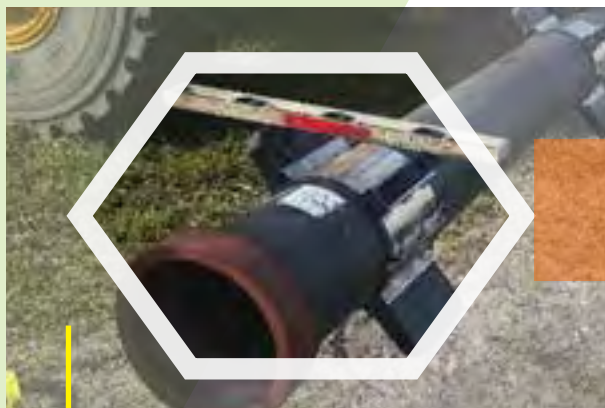
Pipe Spacers in Place for Casing Installation
