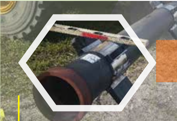
Pipe Spacers in Place for Casing Installation
