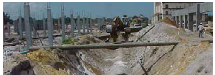
Rosemary Avenue utility relocations underway, while simultaneously constructing the vertical elements of CityPlace.
