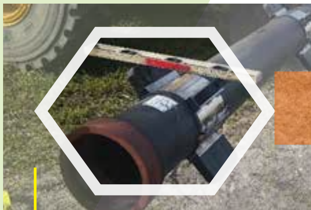
Pipe Spacers in Place for Casing Installation
