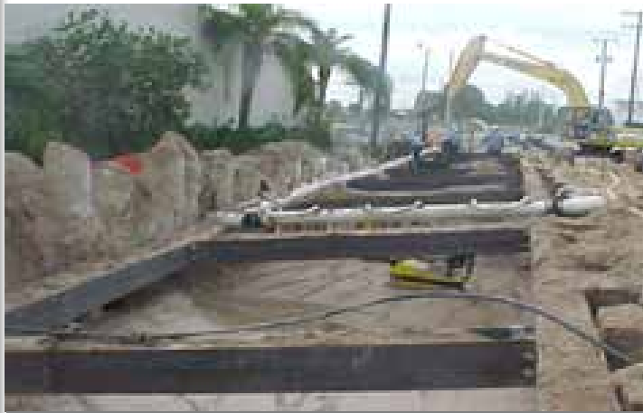
Renaissance 72" Aluminized Steel Pipe (20' deep)
