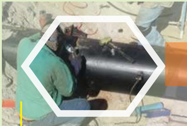
Welding Pipe Casing
