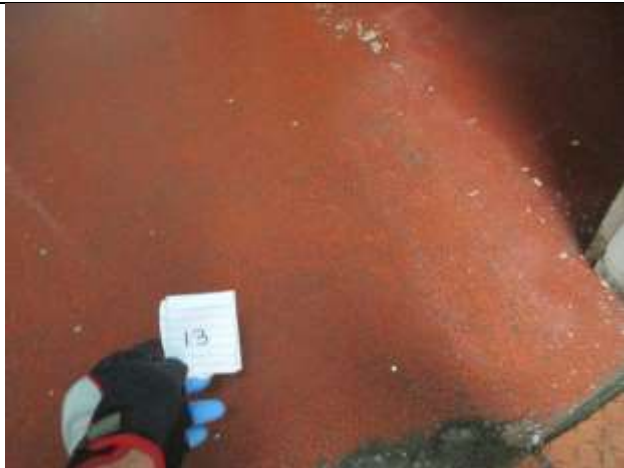
HA 13- Red Rolled Sheet Flooring and Glue
