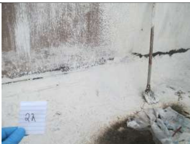
HA 22- Built-Up Bituminous Roofing Material at Flashing
