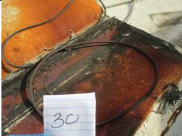
HA 30- Black Mastic on Air-Conditioning Unit Asbestos Containing Material
