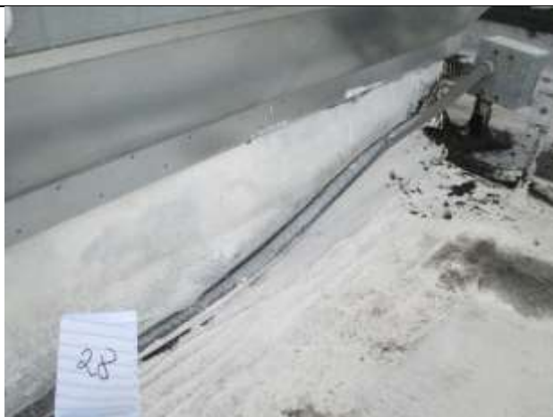
HA 28- Built-Up Bituminous Roofing Material at Vent Curbs
