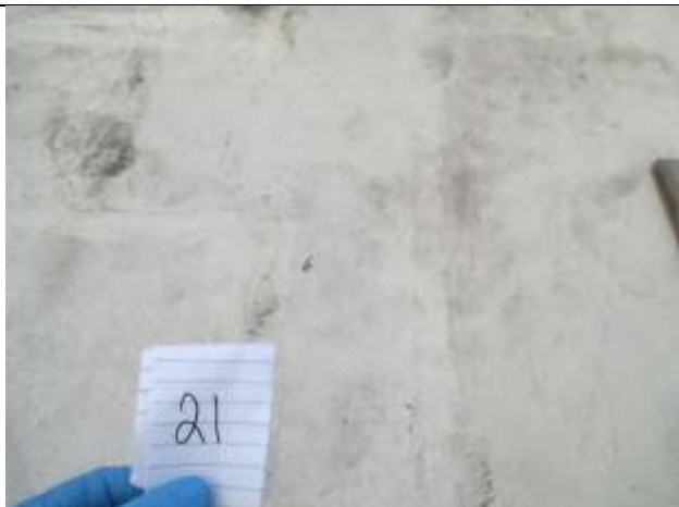
HA 21- Built-Up Bituminous Roofing Material at Membrane
