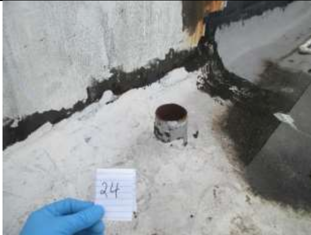
HA 24- Built-Up Bituminous Roofing Material at Deck Penetrations
