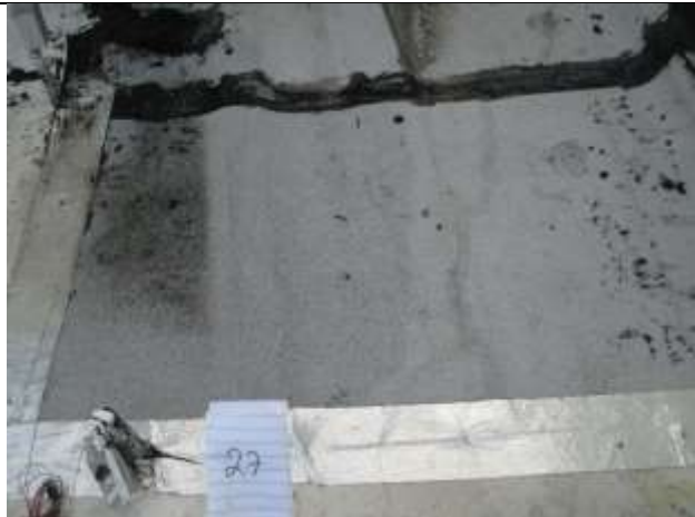
HA 27- Built-Up Bituminous Roofing Material Patch
