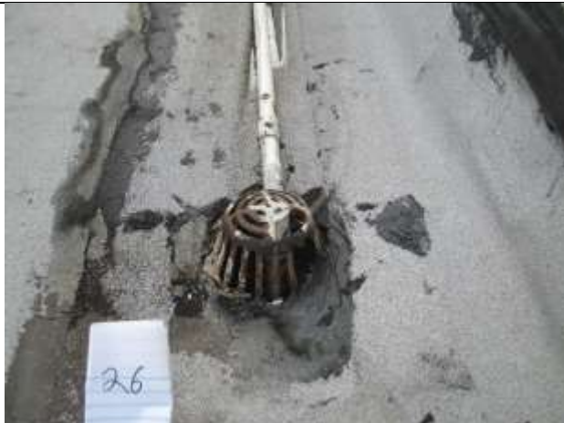
HA 26- Built-Up Bituminous Roofing Material at Drains
