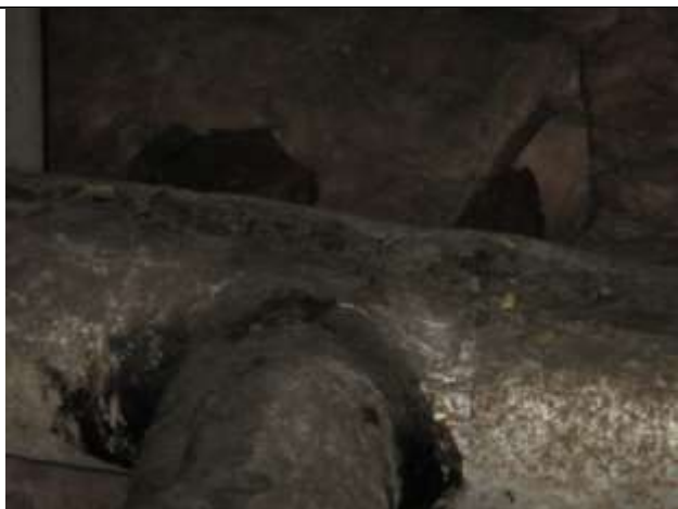
Black Mastic Above Drywall System Ceiling Assumed Asbestos Containing Material
