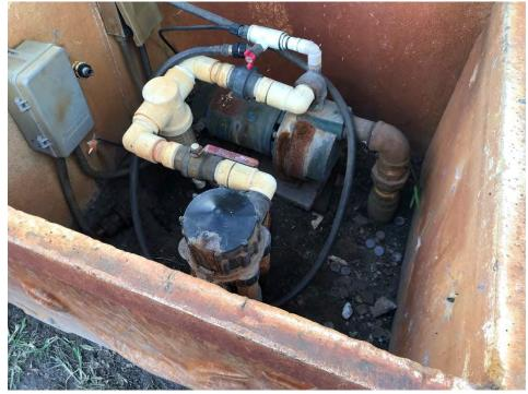
**Photo 9:** View of the irrigation pump located central to the western side of the Site.
