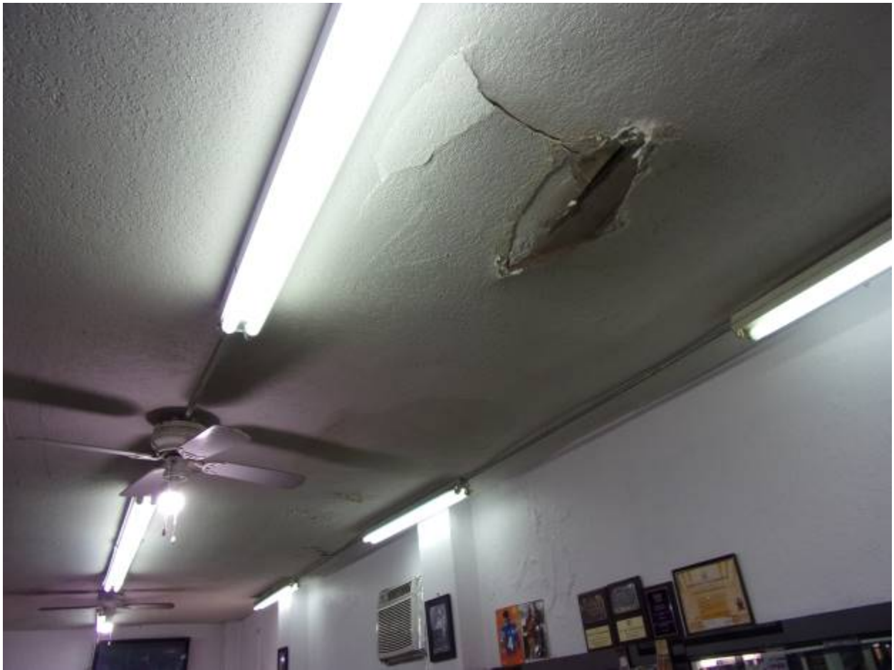
Unit 700 Roof Leak
