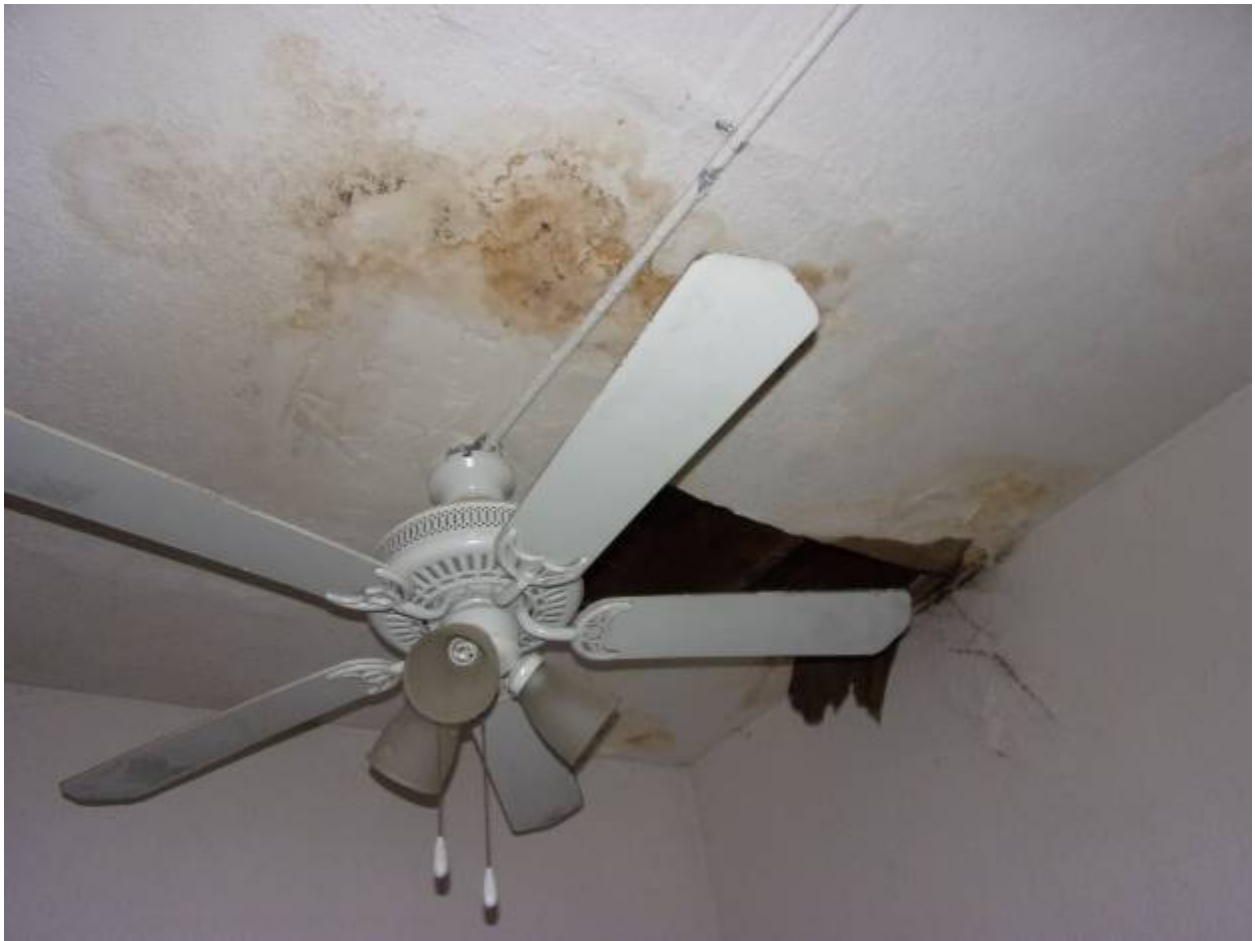
Unit 700 Roof Leak
