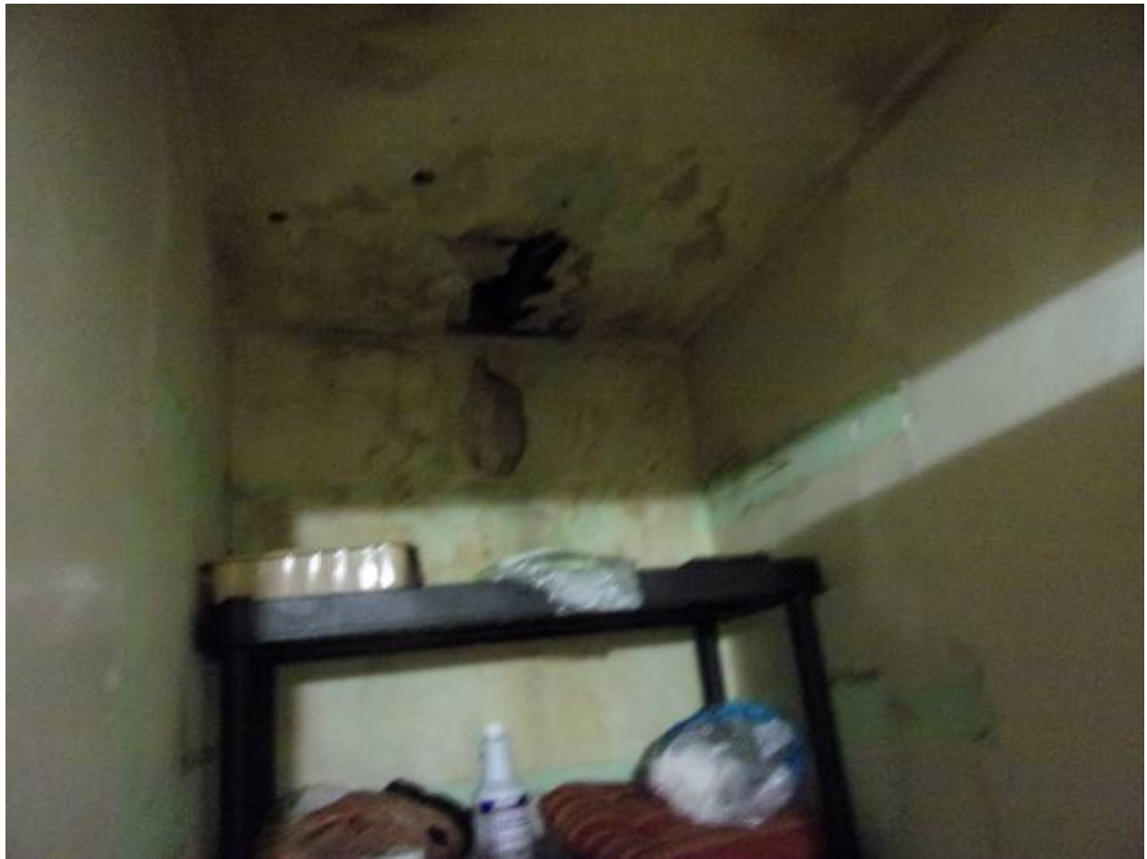
706A Roof Leak
