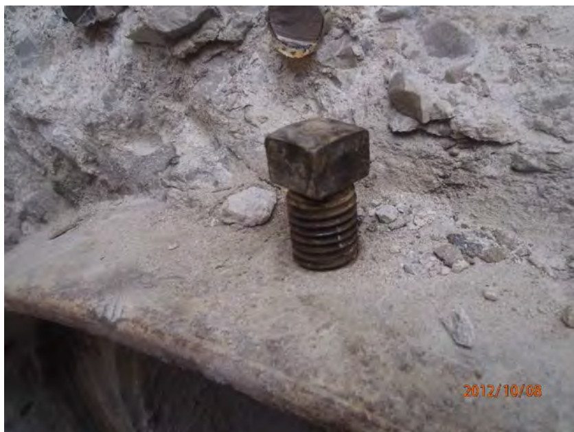
Figure 3: Bell bolt inserted into threaded hole in bell ring
