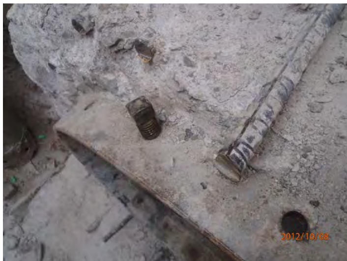
Figure 4: Bell bolt inserted into bell ring
