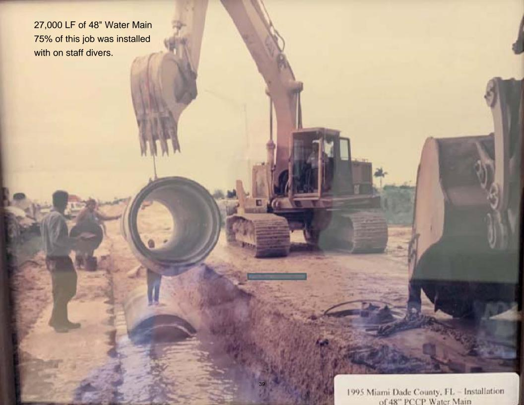
48" Prestressed - Concrete Pipe for Dade County. Trench was precut with trenchers so installing was as much as 400' per day.
